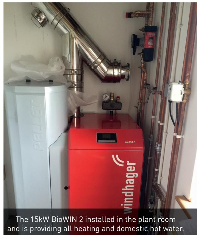
The 15kW BioWIN 2 installed in the plant room and is providing all heating and domestic hot water.
